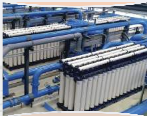
Рис. 2. Ultrafiltration and Reverse Osmosis system for a water recycling plant built by WABAG
